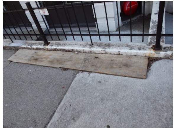
Plank patch, south side Westland
