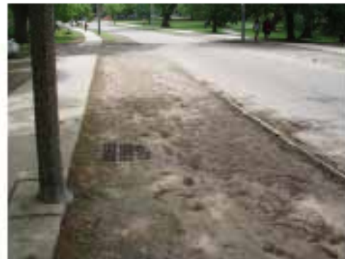
Figure 27 Catch basin inlet demarking old roadway width (two-way traffic) (May 25, 2011)
