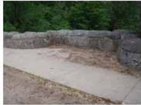
Figure 39 Overlook at Agassiz Road bridge. (May 25, 2011)
