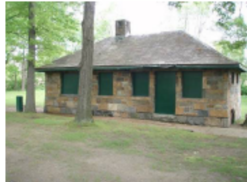
Figure 35 Front (south-facing) side of Duck House (May 25, 2011)
