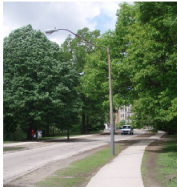
Figure 34 Typical light pole and fixture along Agassiz Road, longer reach arm. (May 25, 2011)
