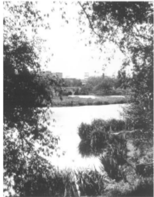
Figure 22 View of Agassiz Road Bridge, circa 1925 (Boston Public Library Print Room)
