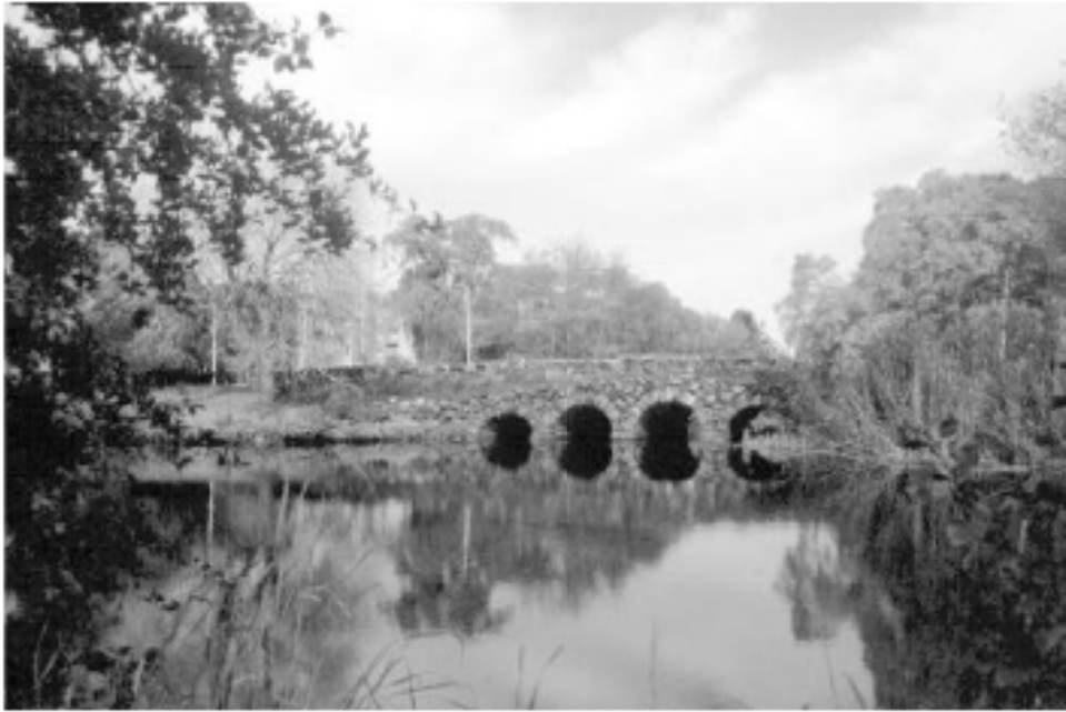
Figure 42 Agassiz Road Bridge immediately following replanting of planting shelf and removal of invasive vegetation in 1989 (Pressley Associates, 1989)
